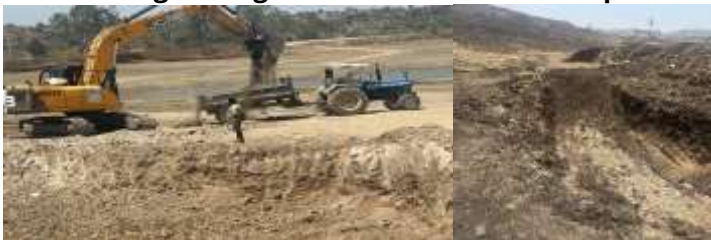
Desilting in Progress and A Section of Deep CCT
